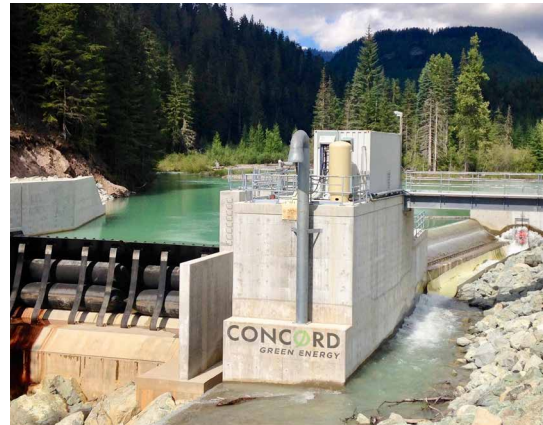
Skookum Power is a 25 MW run-of-river hydro-electricity project that will deliver clean renewable electricity to BC residents.
